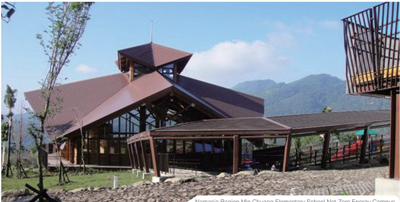
Namasia Region Min Chuang Elementary School Net-Zero Energy Campus (Source: Taiwan Environmental Information Center)
