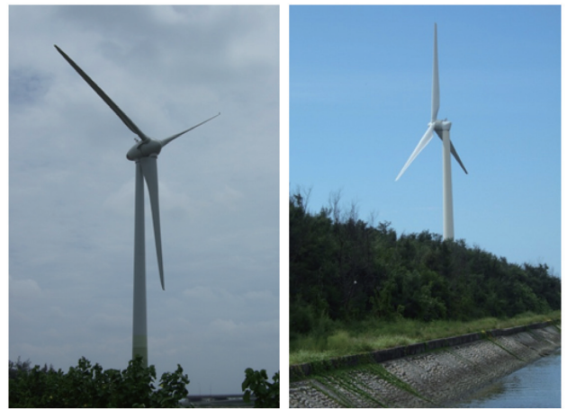
Figure 3-7. Gearless wind turbines installed in R.O.C. (Source: ITRI)
