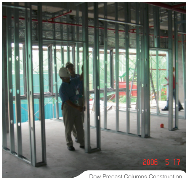
Dow Precast Columns Construction
