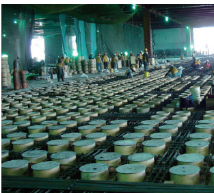
TSMC FRP System Plates
