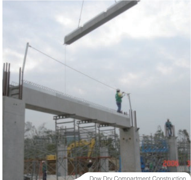
Dow Dry Compartment Construction
