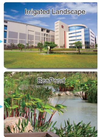
TSMC Rainwater Recycling System (Source: Green Factory Label, 2013)
